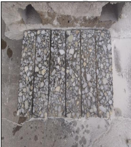
132 FIG. 2: Coatings laying
