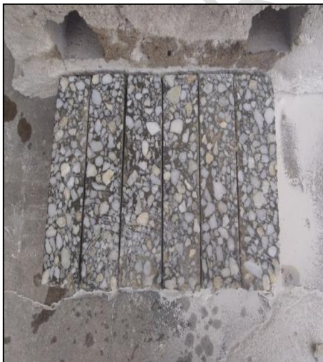
132 FIG. 2: Coatings laying
