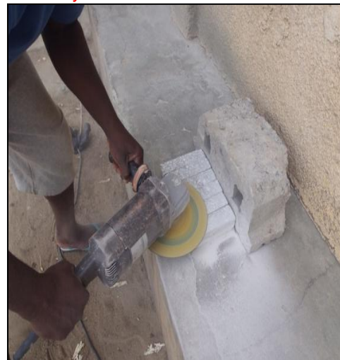
133 FIG. 3: Sanding operation
