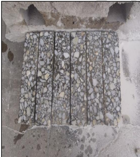
133 FIG. 2 Coatings laying
