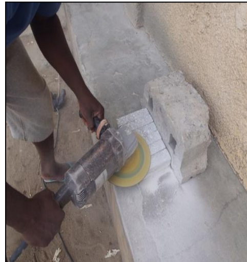
134 FIG. 3 Sanding operation
