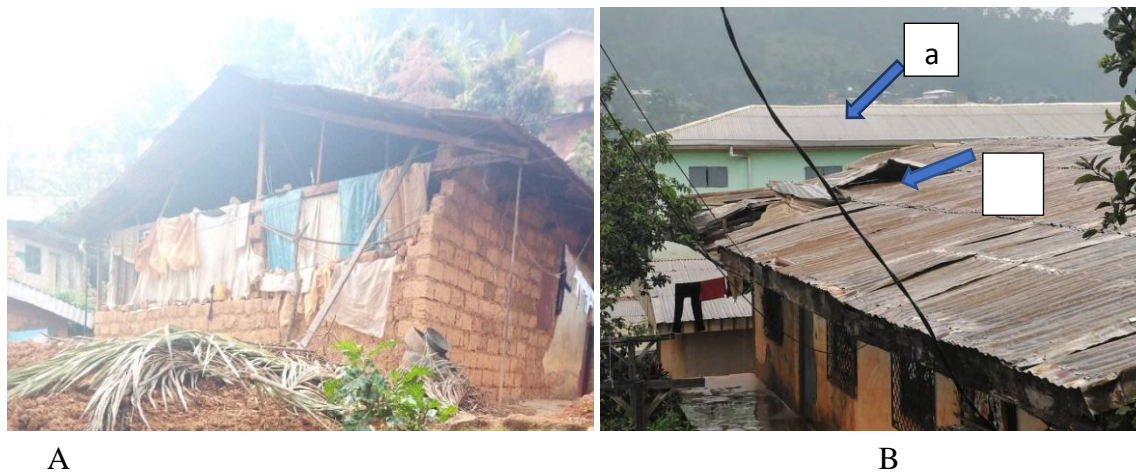
Plate 1A: House built with mud block and rudimentary materials in Sisia Quarter
