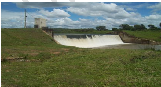
Figure 1: Pictorial View of Unilorin Dam
