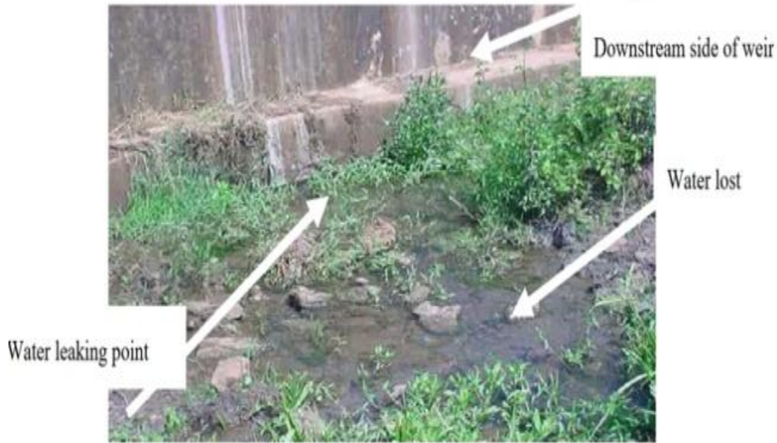
282 Figure 4: Leakage on River Diversion structure
