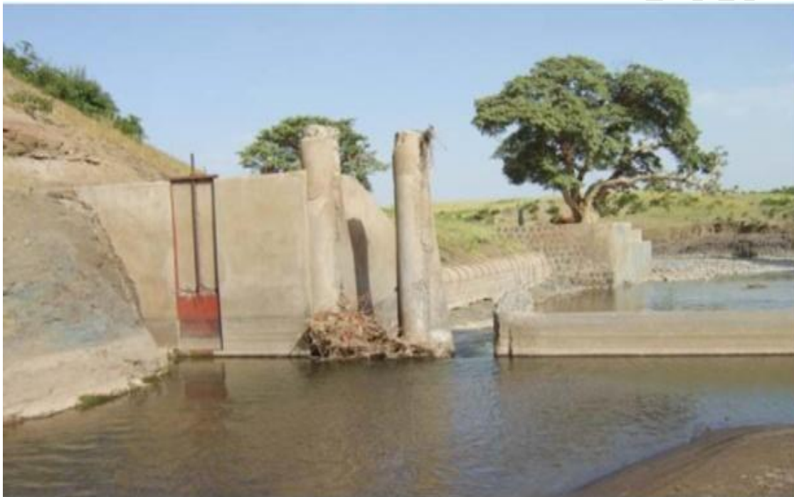
280 Figure 3: Part of River Diversion head work
