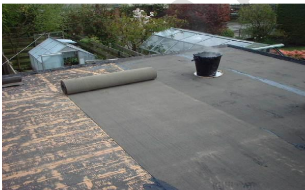
Plate 2: Moisture proofing using bitumen
