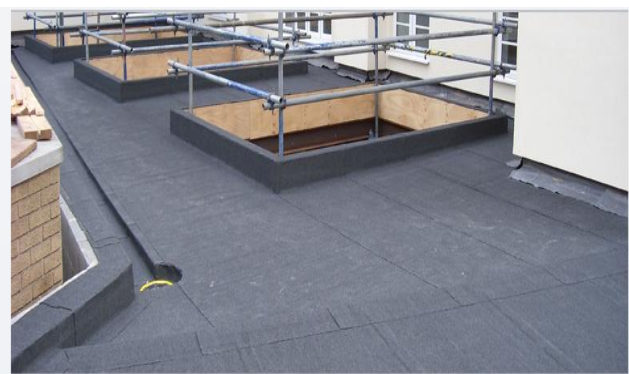
Plate 3: Moisture proofing using asphalt
