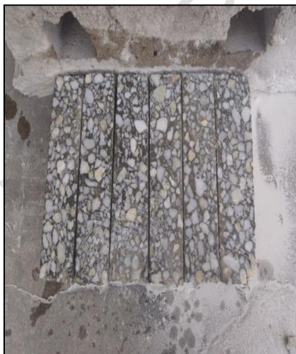
130 FIG. 2 Coatings laying
