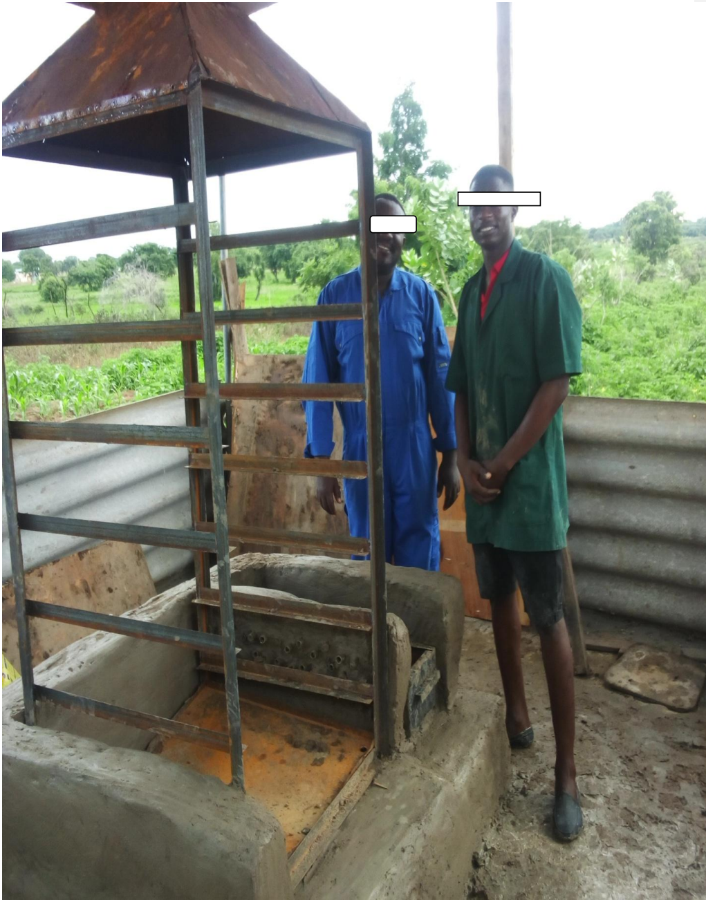
Plate 1: Kiln Wall under Construction
