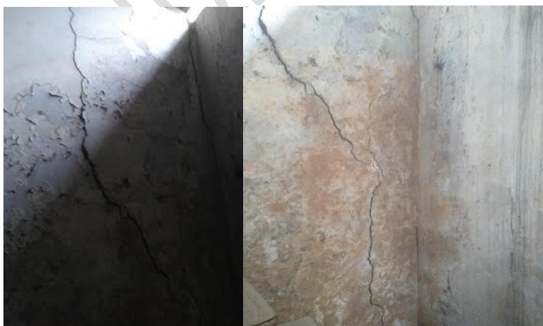
238 Plate 1: Cracks as a result of settlement of foundation
