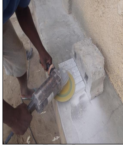
Fig. 3: sanding operation
