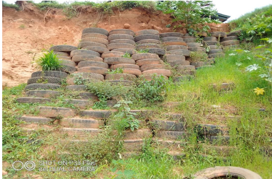
Figure 3: Embankment constructed by the use of tyres Source: Fieldwork 2020
