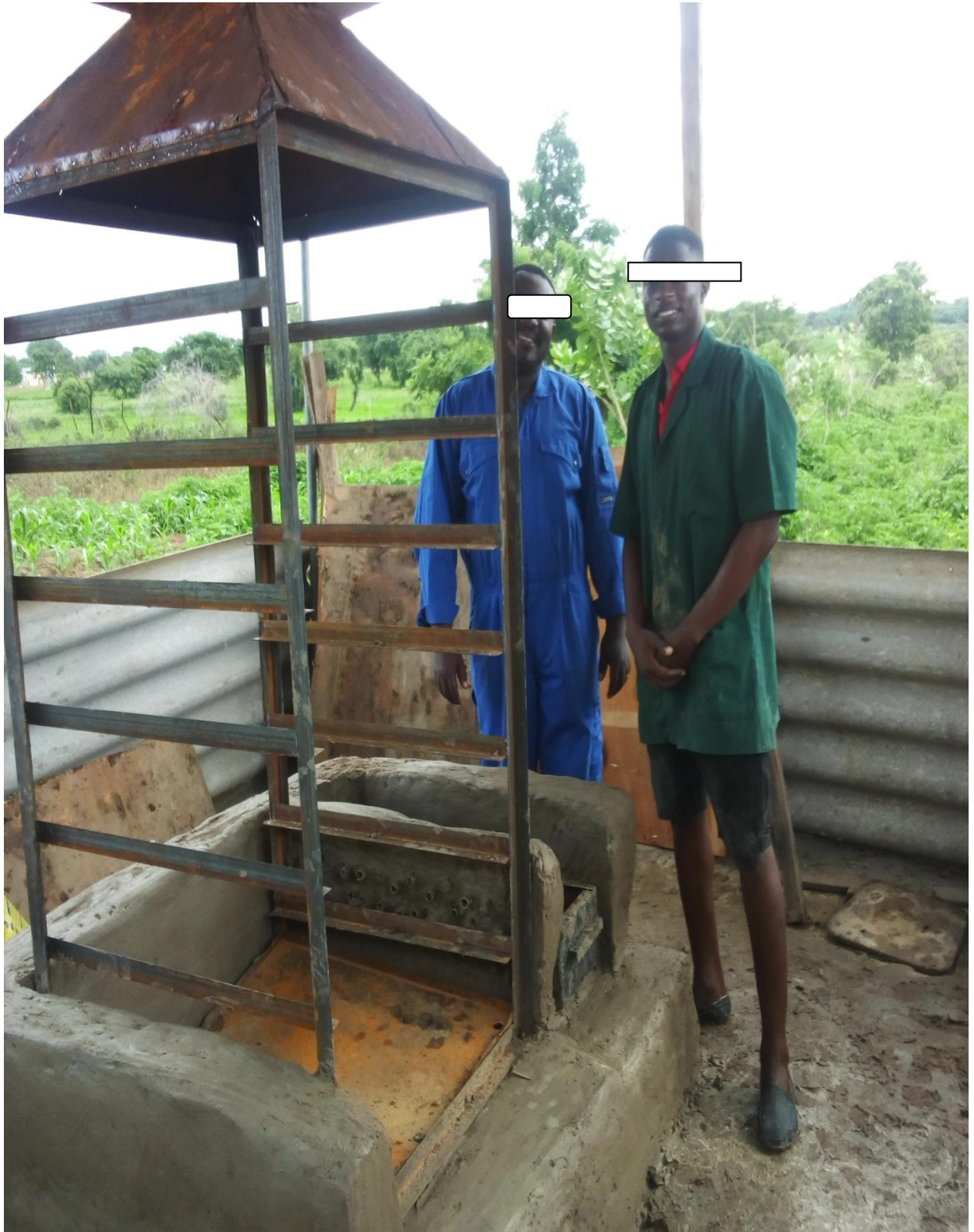
Plate 1: Kiln Wall under Construction
