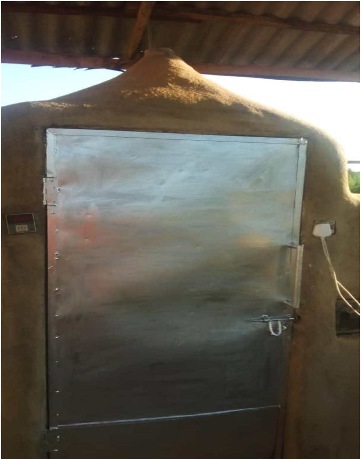
Plate 2: Electrical Fish Smoking Kiln Structure.
