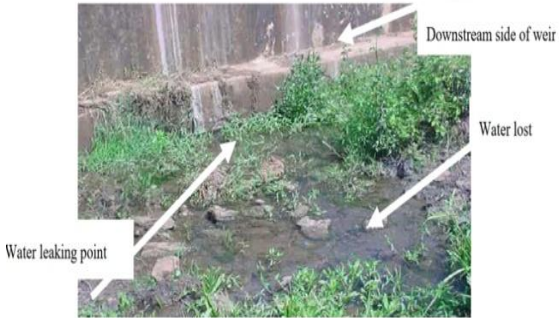
283 Figure 4: Leakage on River Diversion structure
