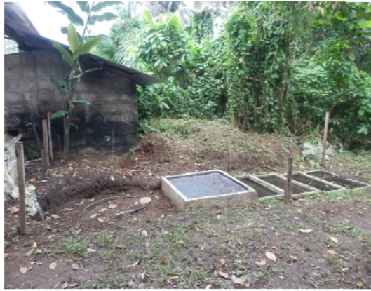
Figure 3. Biogas technology project in Malvar
