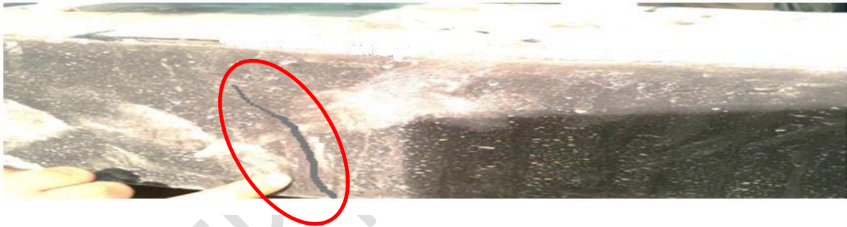
Fig.10. Failure mode of sleeper S 10 under static load on rail seat section
