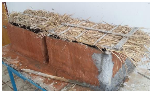
Fig. 5: Finally covering the structure with straw materials
