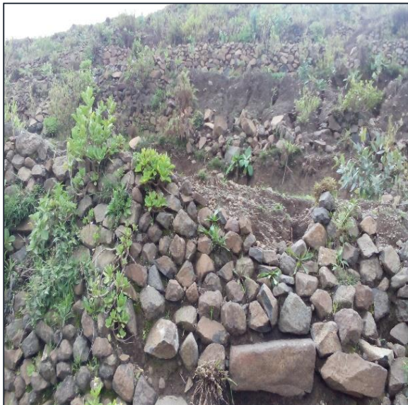
Figure 5 Collapse of terraces due to single line stone placement, no buffer zone and not support with biological SWC practices
